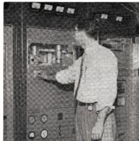
KFEL-TV Denver's Chief Engineer Rhea Cunningham looks over the station's new DuMont 25 kw high power television transmitter before it was shipped from DuMont Labs, Clifton, N. J. KFEL-TV will use the equipment (DuMont's first of its kind) to increase power to 100 kw.
